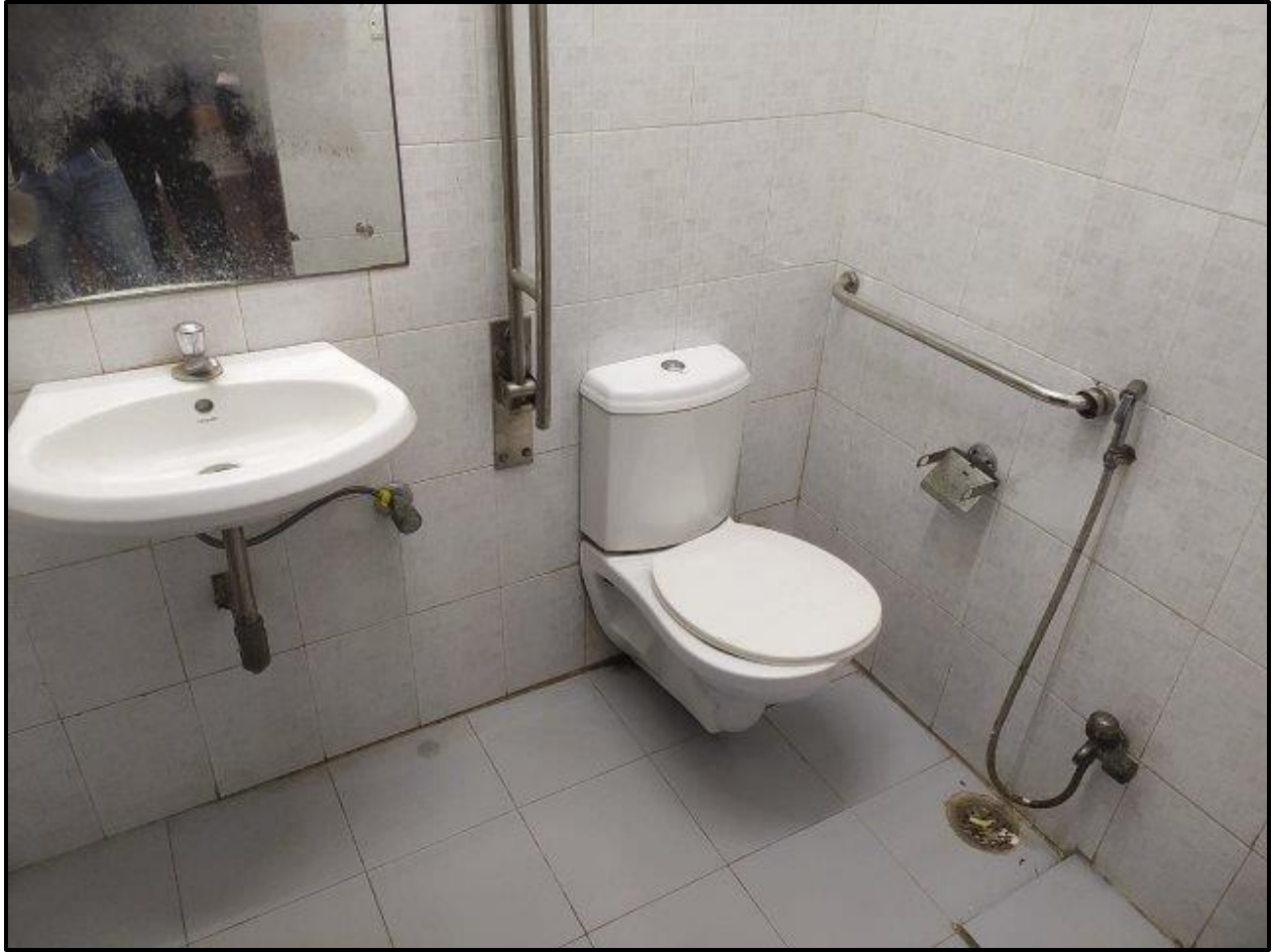
Figure 24: Differently Abled Washroom
