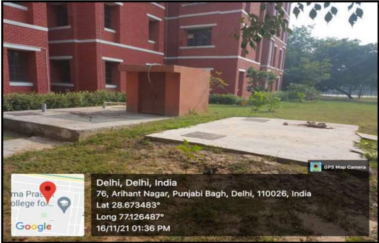
Figure 8: Rain Water Harvesting Tank with storage capacity of 50000 Litres and 3 Layer bore Filer media
